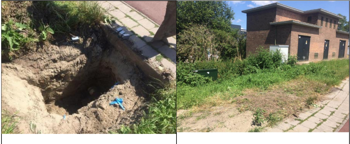
Figure 21 Surroundings of the measurement set-up in location M5
