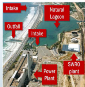
CARLSBAD (SAN DIEGO) - OPEN INTAKE
